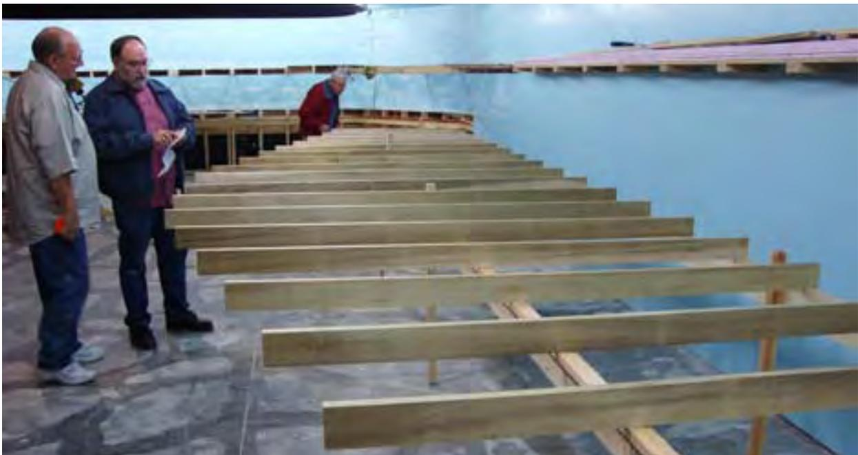
This is where it is all headed: Amarillo Junior Yard bench work temporarily in place. There will be a narrow access aisle between the wall and the yard. The main line will run down the wall side. Our narrowest members will clear up derailments, etc. in this area.
