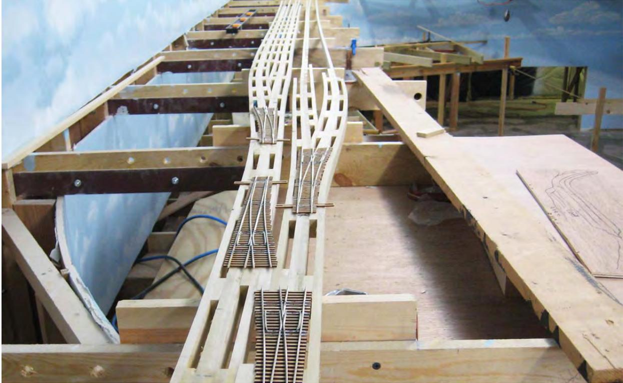
Upper level from the north end. The transition from two lines to four lines is more clearly shown. The turnouts have been placed on the roadbed to show how spline roadbed works with long, flowing paths. The height of the rail may vary, but the vertical transition is also smooth.
