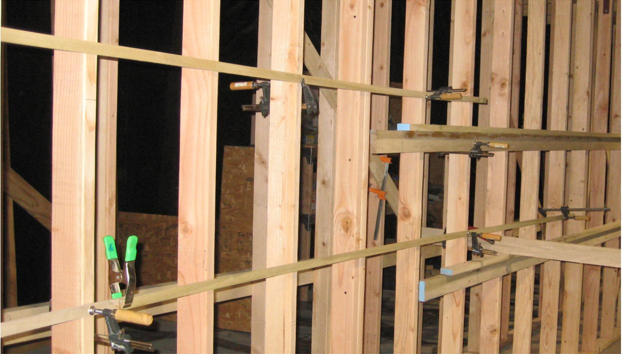
Track level strips coming into Hereford on the upper level and into Panhandle on the lower level. Thjere will not be any L-Girders on the upper level. This one is used for study purposes only.
