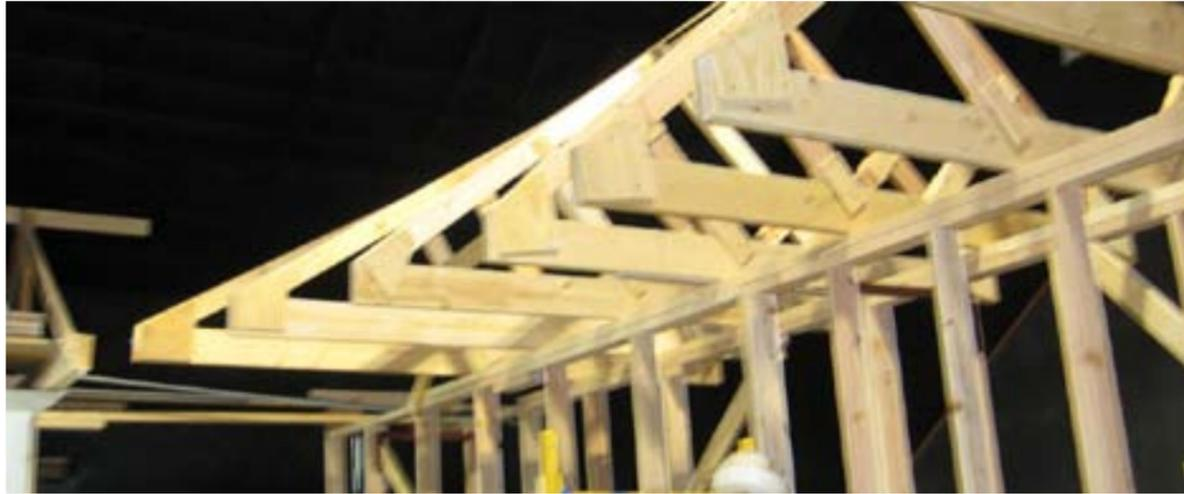
The installed girders over the beginnings of the Canadian yard on the far side and the connections of the staging yard with the northern strip of Amarillo Yard on the near side. Some special girders will have to be built to tie this section of roof girders with those along the south wall.
